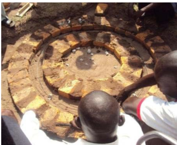
Picture 18: The concrete foundation with metal rings
