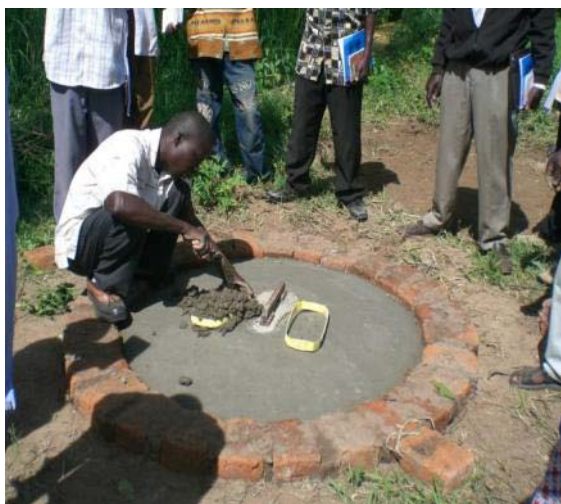
Picture 14: Filling moulds for foot rests on dome slab
