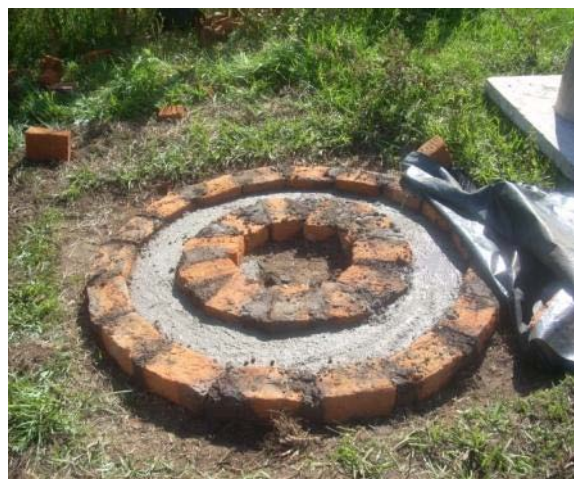
Picture 19: Ring foundation curing
