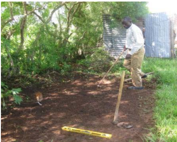
Picture 6: Preparing the ground for slab construction
