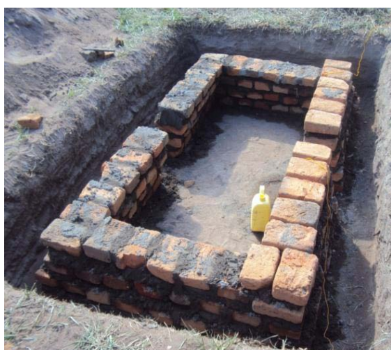
Picture 22: Corbelled foundation for a double stance latrine pit
