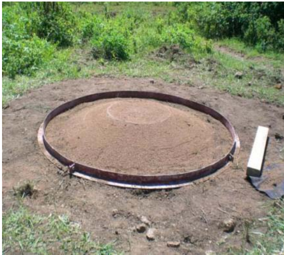
Picture 8: Circular mould with wet sand placed, compacted and smoothed
