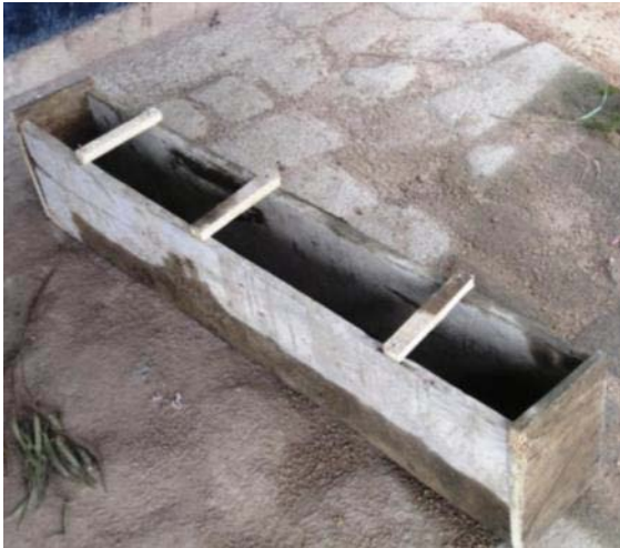
Picture 10: Mould for casting concrete beam for a double stance latrine
