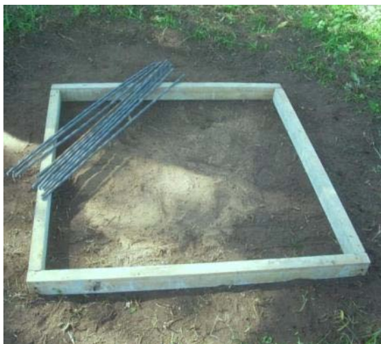
Picture 5: Wooden Mould and reinforcing bars for square slabs
