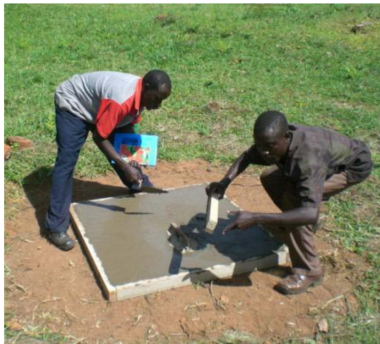
Picture 13: Moulding for a square slab with drop hole mould
