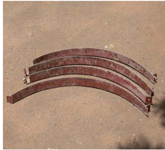
Picture 2: Dome Slab Outer Mould in Knockdown condition
