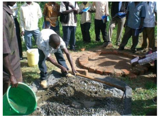
Picture 7: Mixing concrete for slabs
