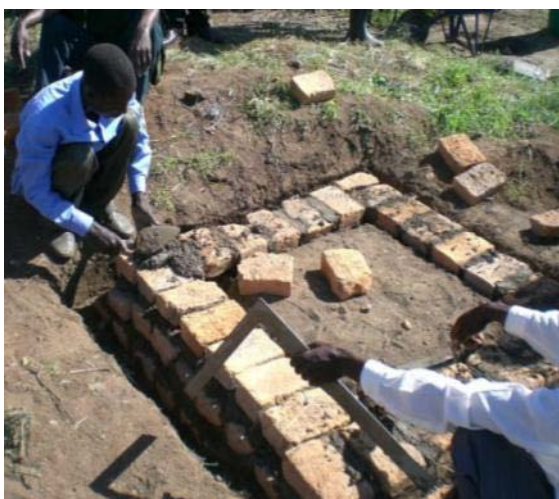
Picture 20: Constructing a brick foundation for a rectangular pit
