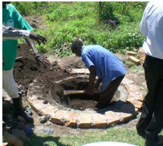
Picture 23: Digging a circular pit within the brick foundation
