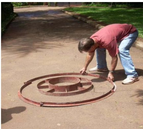
Picture 3: Assembling the outer mould
