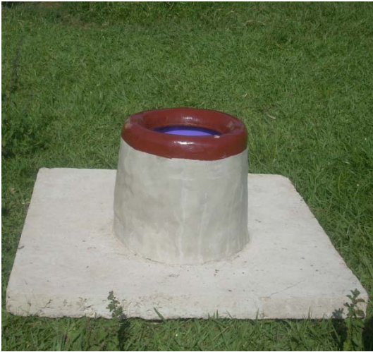
Picture 17 Raised seat on square concrete slab
