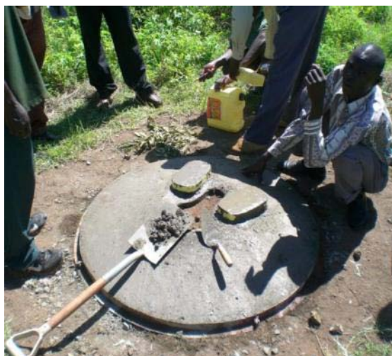
Picture 15: Completing a Dome Slab
